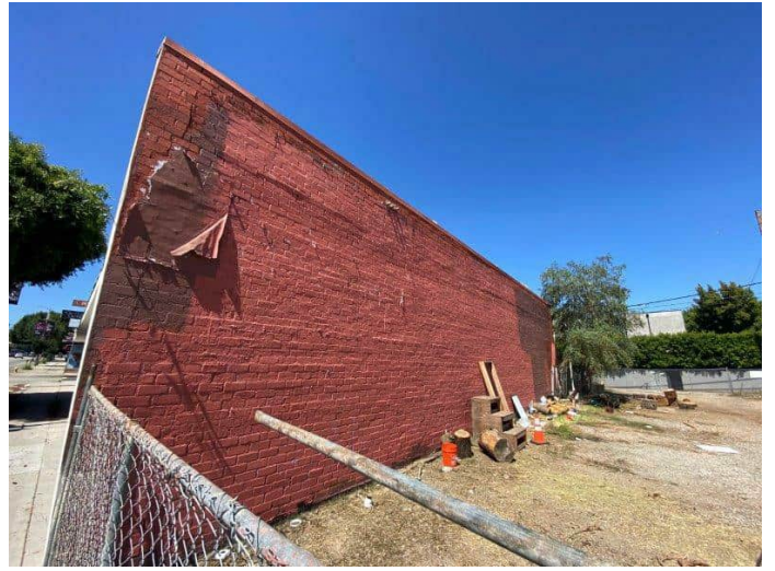
2. Northeast exterior of the building
