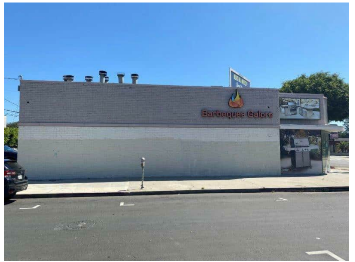
4. Southwest exterior of the building
