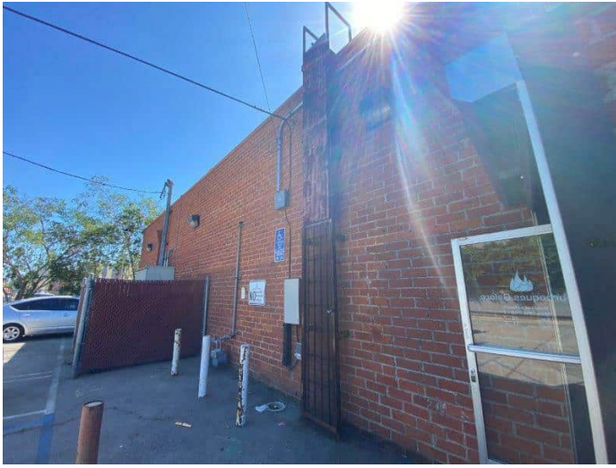
1. Northwest exterior of the building
