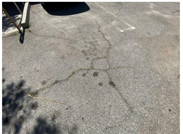
6. Asphalt pavement condition
