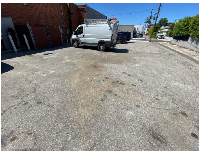
65. Asphalt pavement condition
