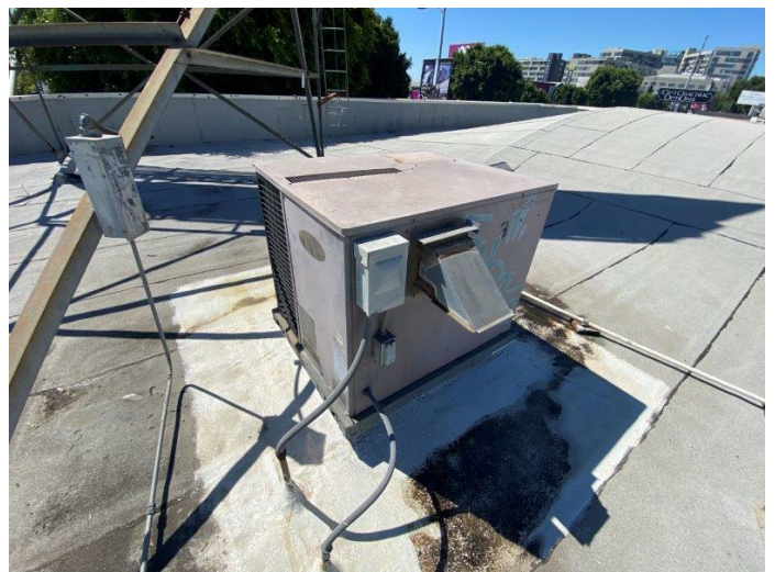
48. Single packaged heat pump
