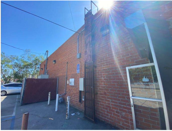
1. Northern exterior façade
