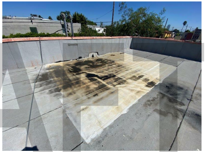
34. Area of recent roof repair
