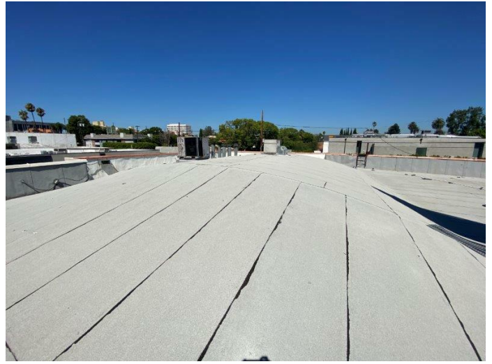
44. View of the roof field
