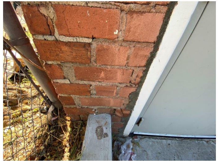
20. Brick masonry condition
