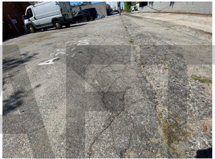
64. Asphalt pavement condition
