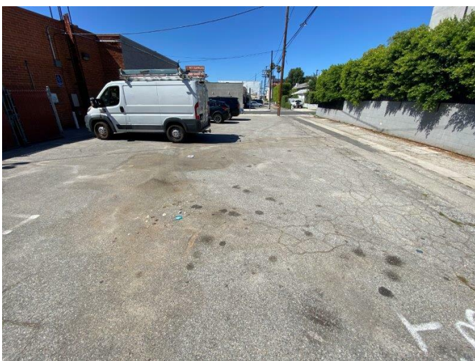
17. Asphalt pavement condition
