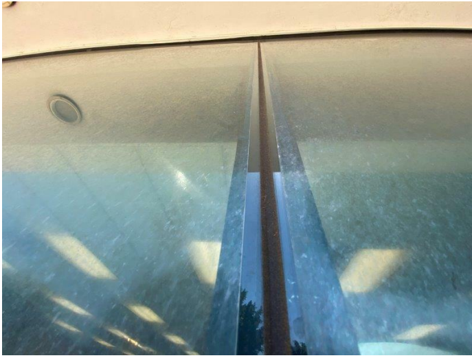
25. Window sealant condition
