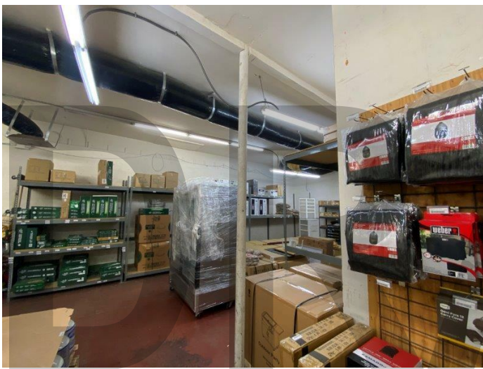
21. Structural component in the warehouse
