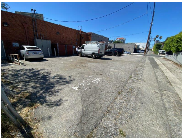
5. Overview of the asphalt paved parking area
