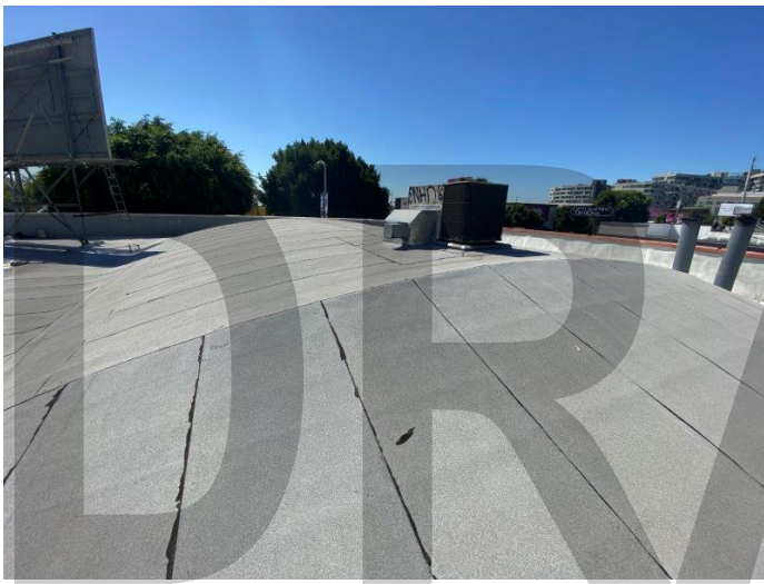
33. View of the bowed roof
