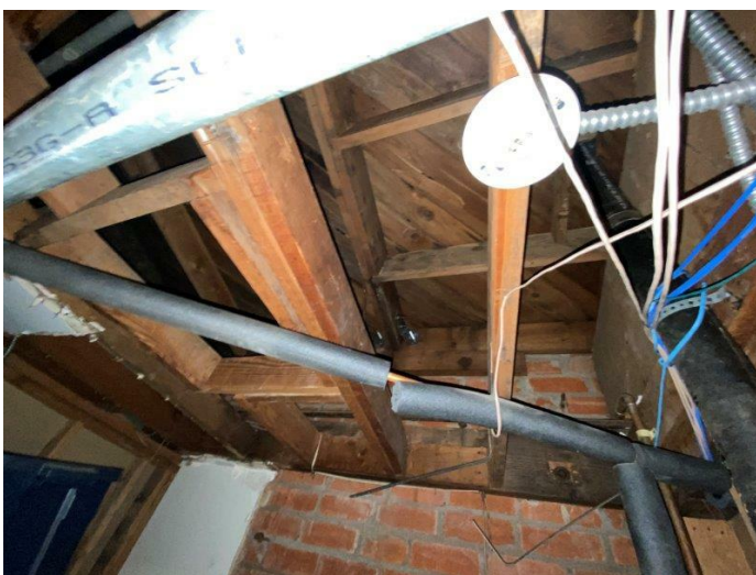
23. Roof framing elements
