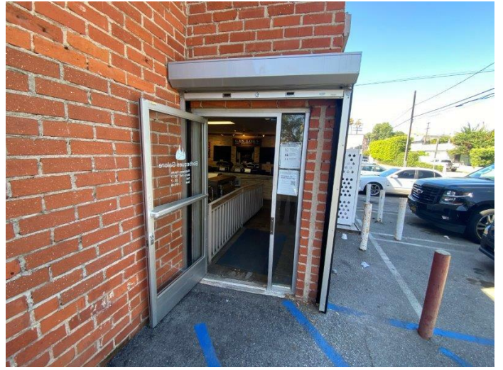
26. Secondary entry storefront system
